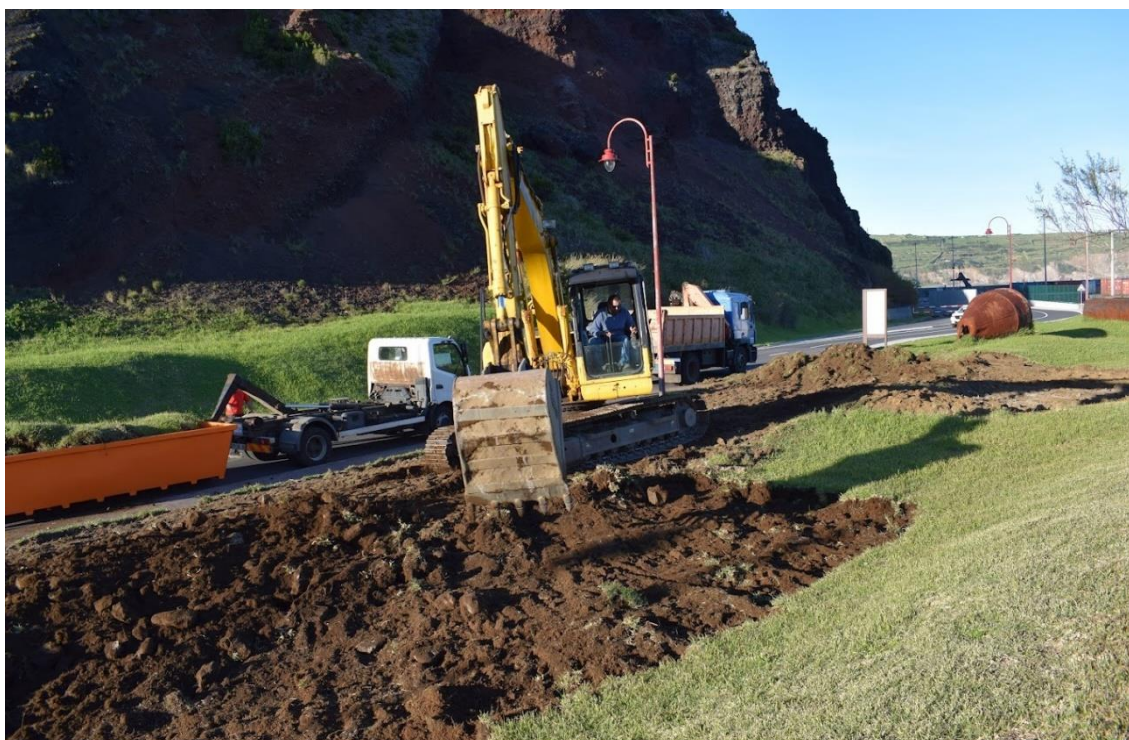
Figure 1 - Heavy Machinery works in Monte da Guia Intervention Area
