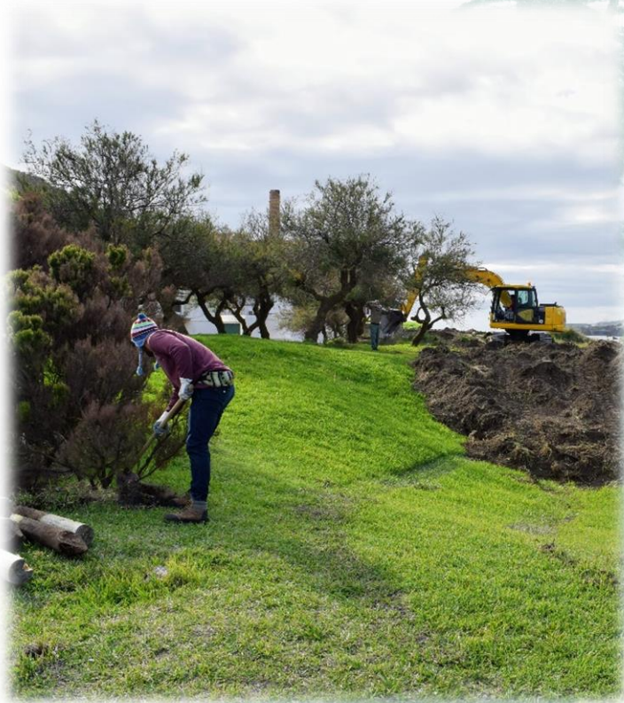
Heavy machinery and manual IAS control works
